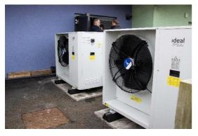
UK boiler manufacturer Ideal provided two Ecomod air source heatpumps for installation at Ysgol Tir Morfa as part of a field trial. The equipment uses air temperature and electricity to generate heat in place of a gas boiler. The efficiency of the system will help lower carbon emissions and costs compared to a traditional boiler. In addition to the
